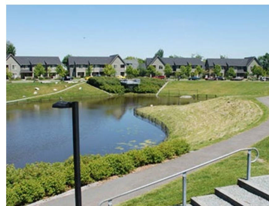
6 STORMWATER RETENTION POND
