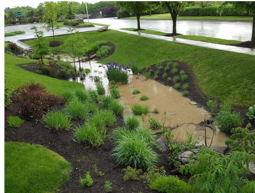
1 RESIDENTIAL STORMWATER DETENTION
