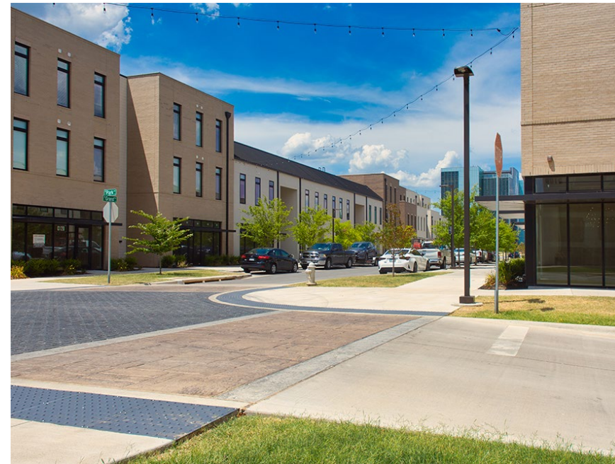
1 RAISED PEDESTRIAN CROSSING
