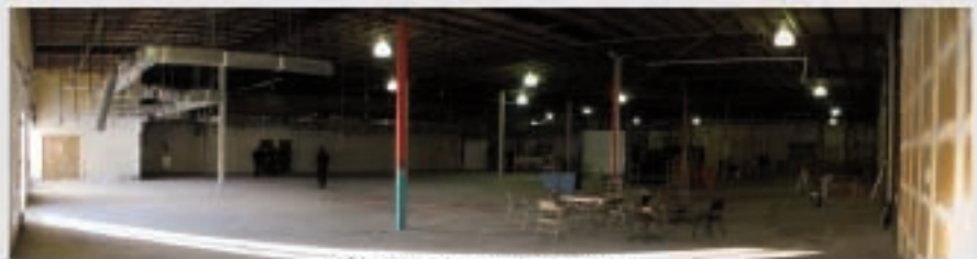
1907 Carpenter during renovation Photo taken by Polk Co EMA staff
